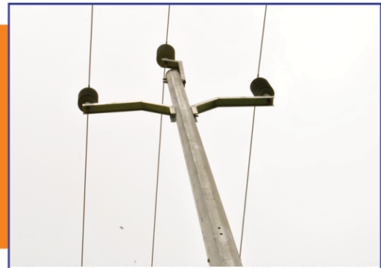
33 KV Transmission Line
